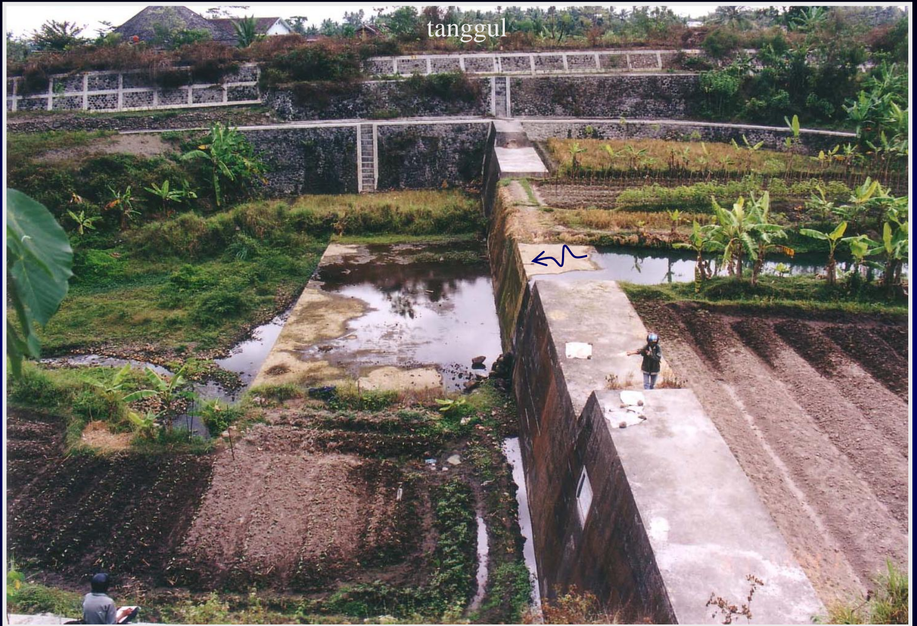
Consolidation dam BO-C2B
