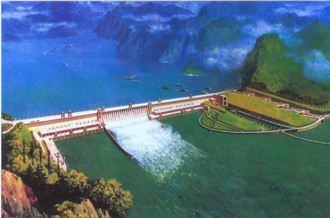
Fig. 3. Artist's impression of the completed dam showing the ship lift and ship lock on the righthand side of the picture
