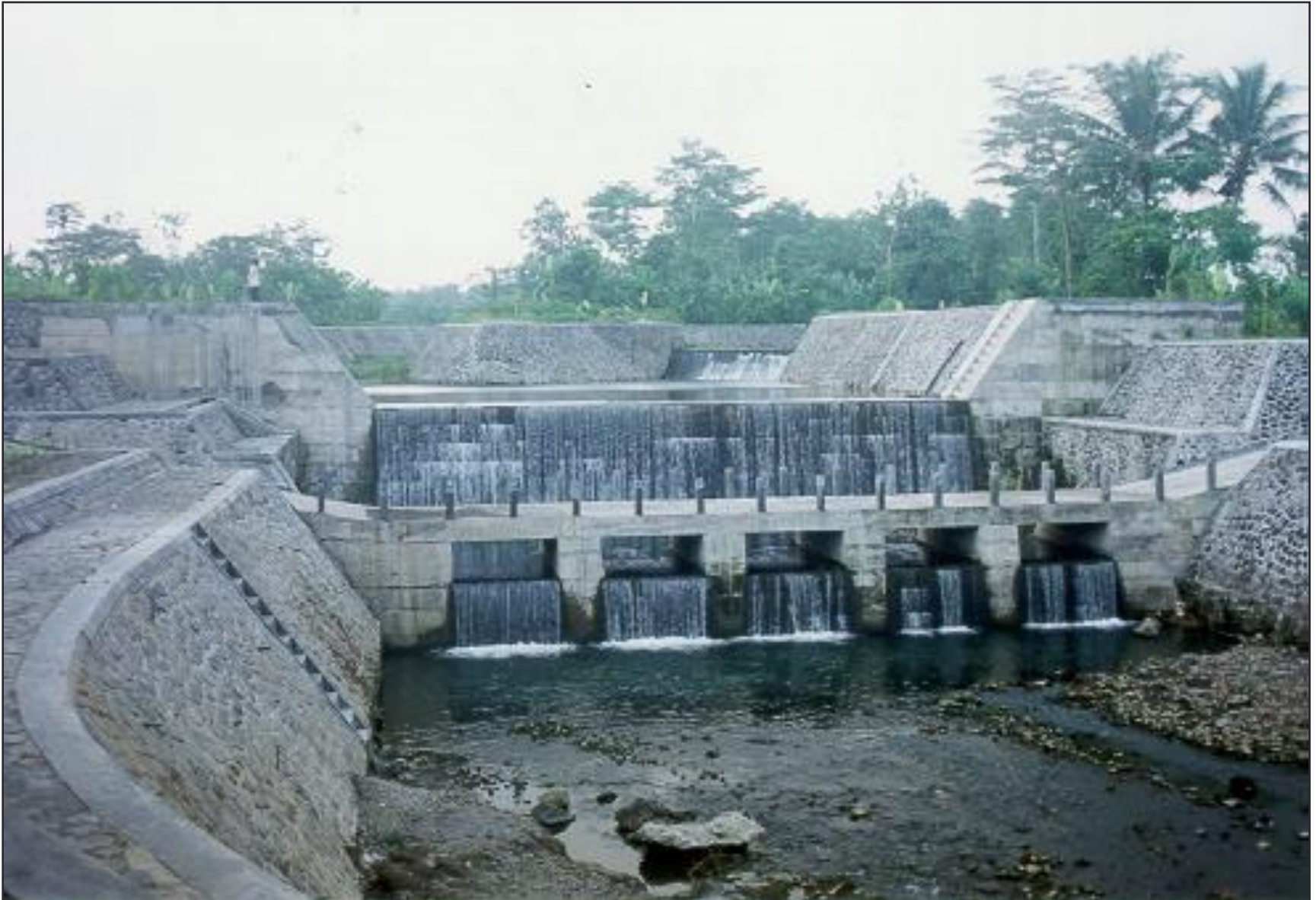
Cannal works Sungai Boyong
