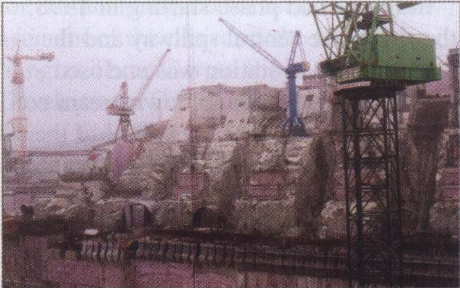
Fig. 16. Dam and north power station under construction
