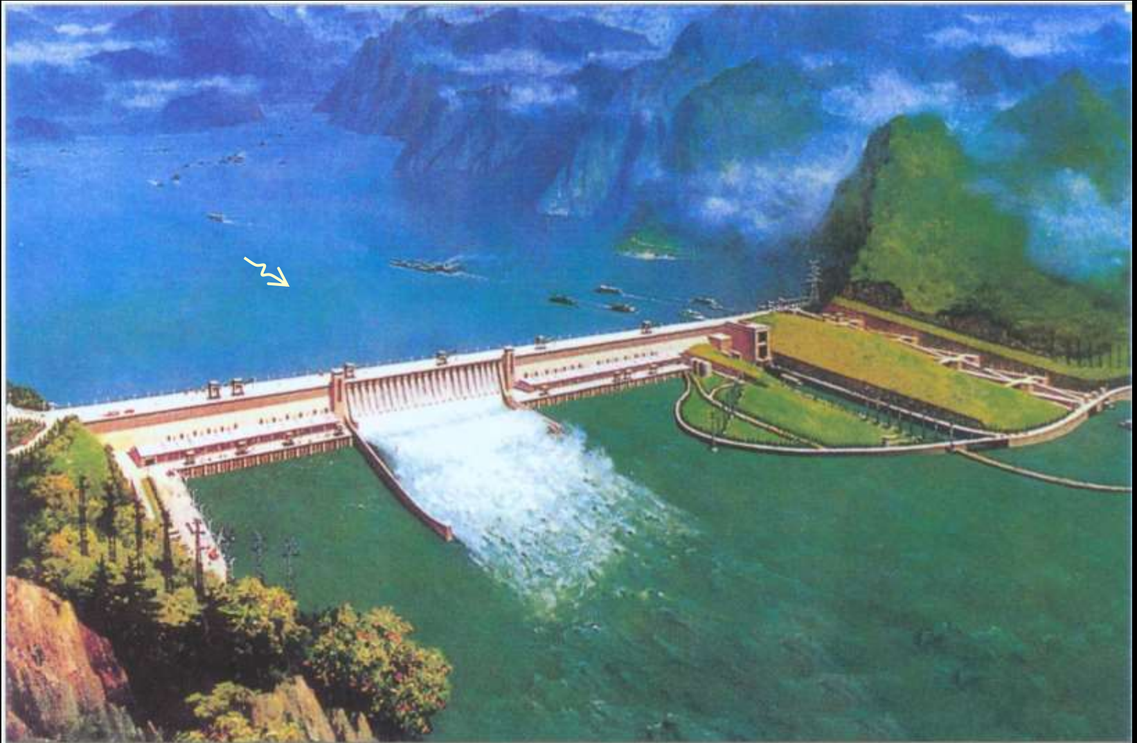
Fig. 3. Artist's impression of the completed dam showing the ship lift and ship lock on the righthand side of the picture
